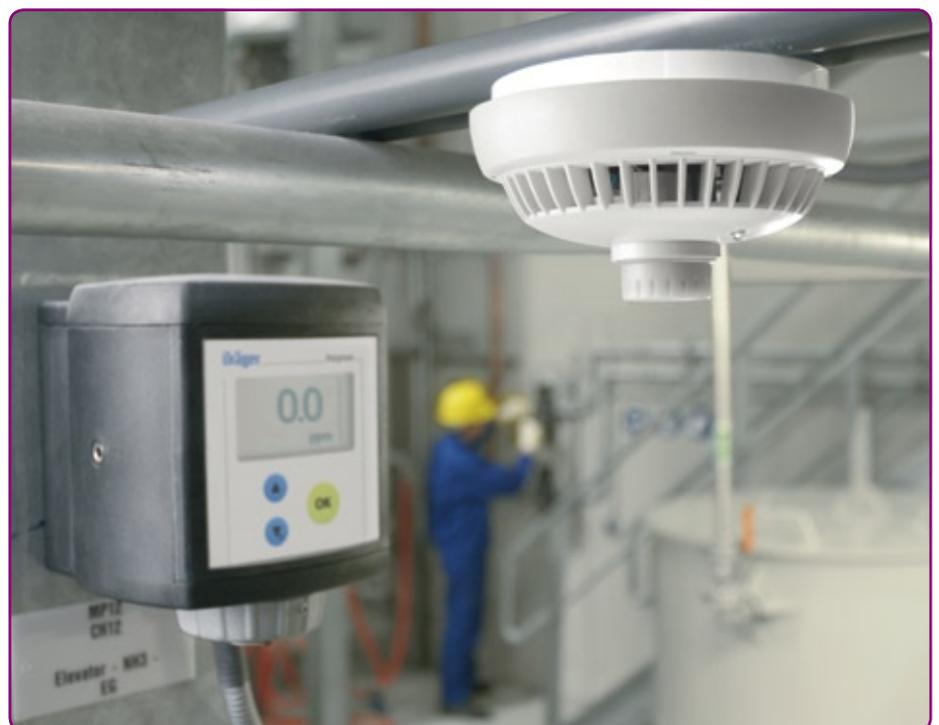
Classic punctiform fire detectors identify imminent danger through the detection of smoke. They are used in offices and in industry. However, these alarm generators do not necessarily suit every condition. In environments where fog appears regularly, for instance, fires will need to be identified by another method rather than smoke detection.
